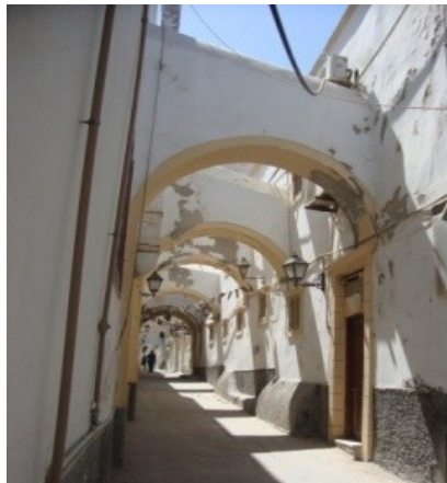
Figure4: The corridor area maintains the varying air pressure (high and low). The gallery is associated with cooling air currents within the space.
